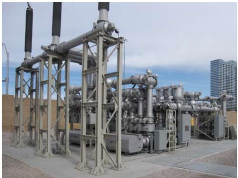
The undamaged 230-kV GIS equipment was protected by the firewalls.
