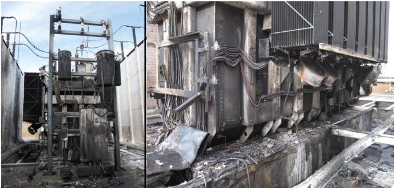
Front and side views of the burned unit with the tertiary structure beside it, although all the equipment on this structure was destroyed, NV Energy was able to repaint and put the steel structure back in service.
