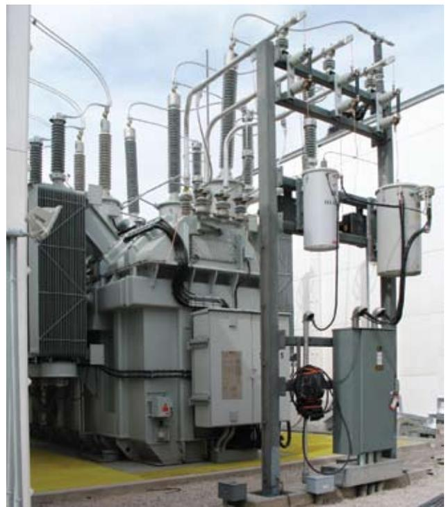
The 230/138-kV autotransformer tucked between the two ceramic panel firewalls before the fire.
